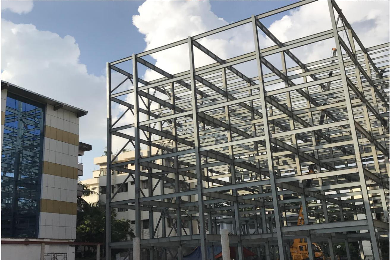
7-Storeyed (95000 Sft) Pre-fabricated Steel Hospital Building at Police Central Hospital, Rajarbagh, Dhaka.
